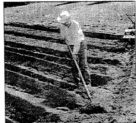
Photo 4-33: Step 4 — Use furrower blade attachment to make irrigation trenches at the ends of each row.
